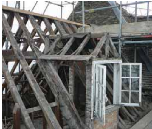
The old timbers on the north wing roof, bridging Merton Hall and the School of Pythagoras, needed extra support from new rafters and ceiling joists.
