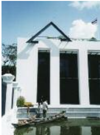
North end of the west elevation
